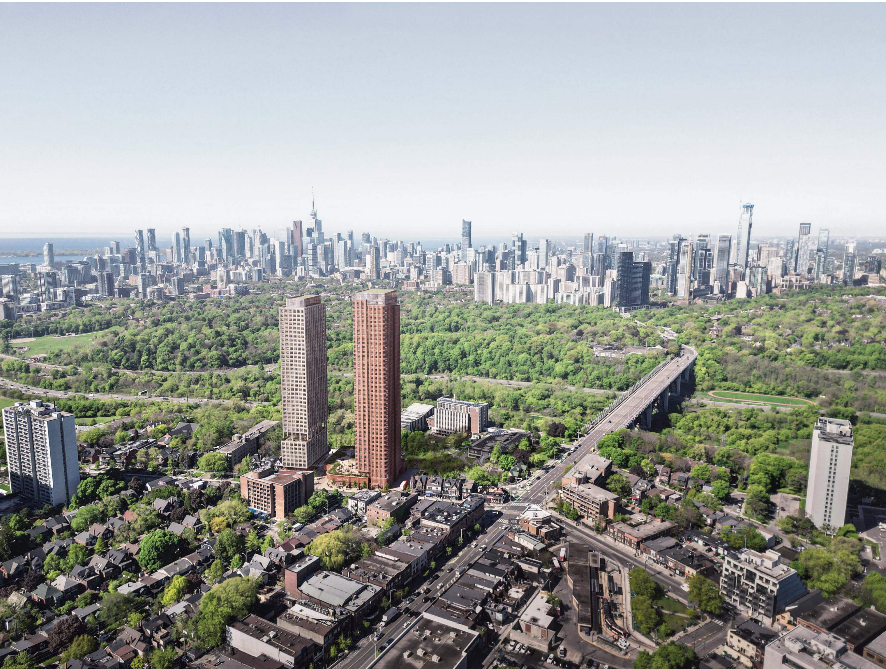
AERIAL VIEW OF PROJECT SITE LOOKING WEST
